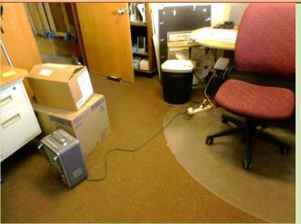
Electrical safety. Portable heater, high electrical load (1850W) ran through power strip. Electrical power strip rated for 1800W continuous use rating. Potential exists for heater to exceed power strip manufacturer's recommendations and create electrical fire. This power cord arrangement also presents a tripping hazard for entrants into this space. Re-route heater and direct to wall plug-in to remove hazard for electrical fire.
