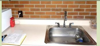
GFCI outlet needed. Outlets close to water sourcess must be GFCI to protect from shock hazards. Work order submitted.
