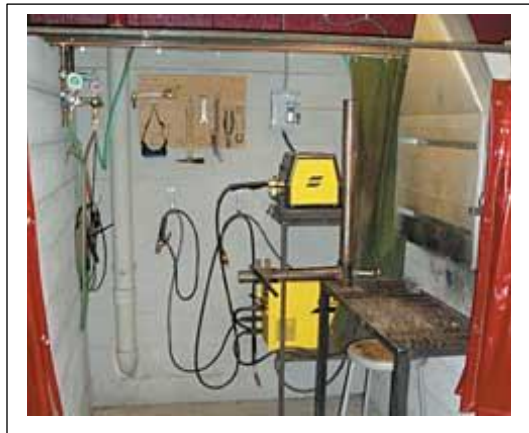
Fixed Exhaust System
