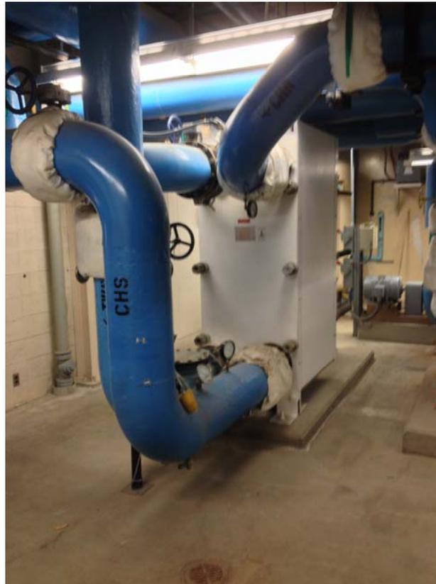
Free Cooling Plate & Frame Heat Exchanger
