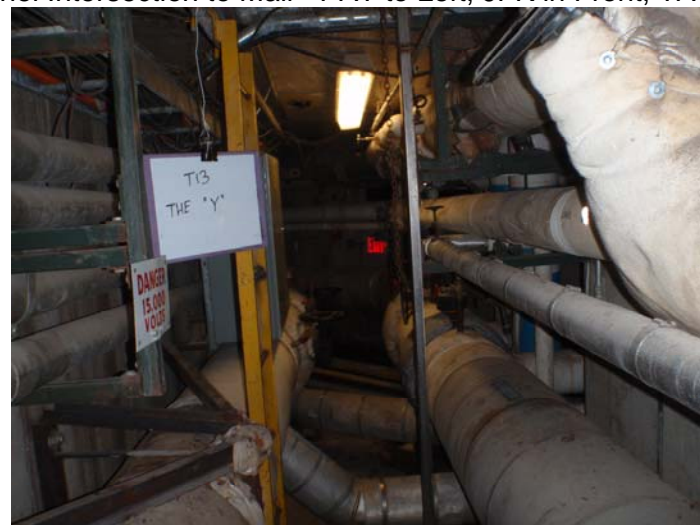
Tunnel "Y" Intersection to PUB Branch (to the right)
