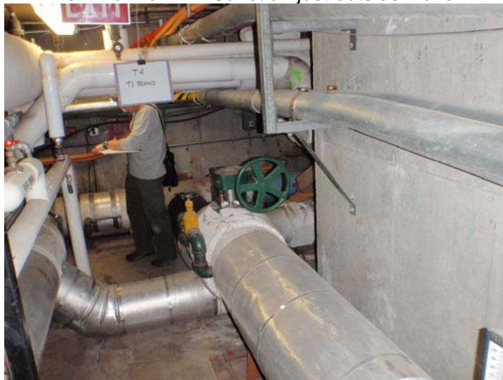
West Tunnel - Intersection to HPE Complex
