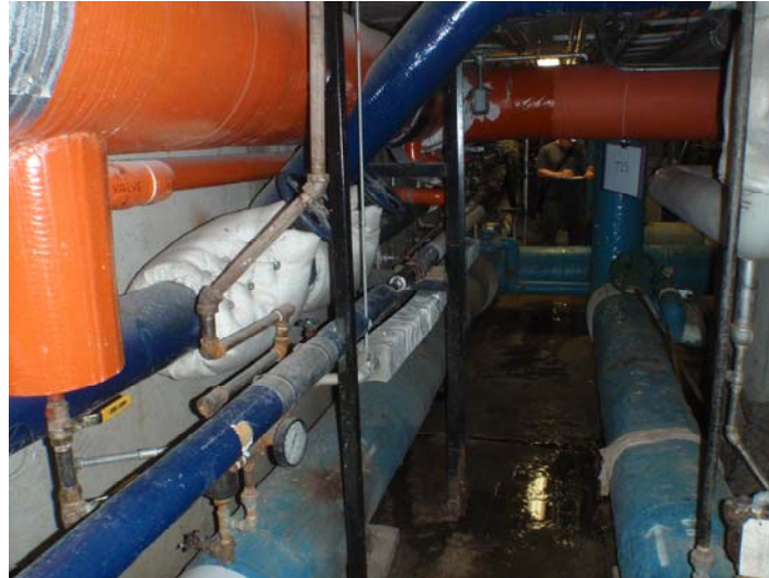
E-W Tunnel Intersection at Branch to Art Complex
