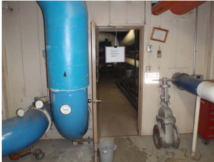
Utility Tunnel Entrance at Rozell
