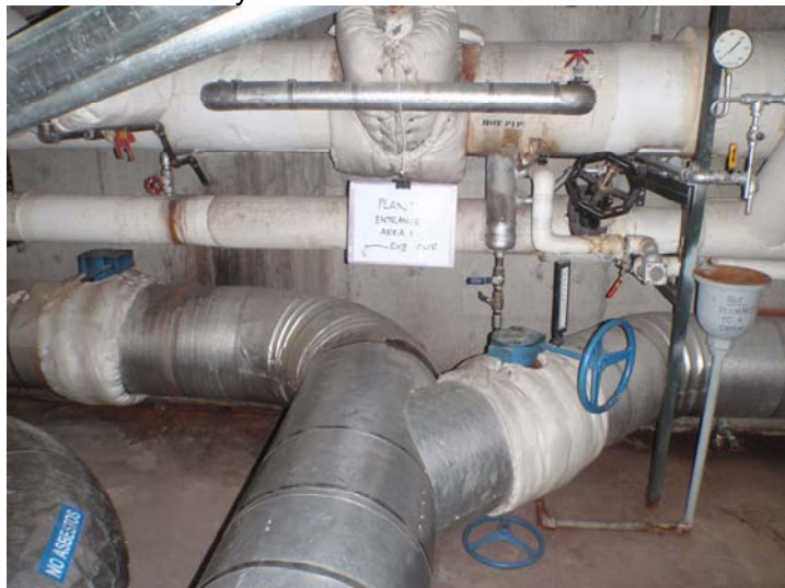
Main Tunnel E-W Junction just outside Rozell
