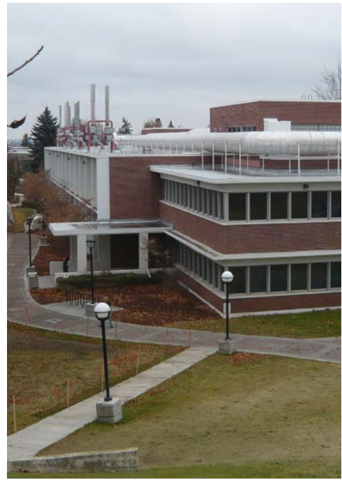
Figure 2.d EWU Science Building Roof top mechanical ductwork
