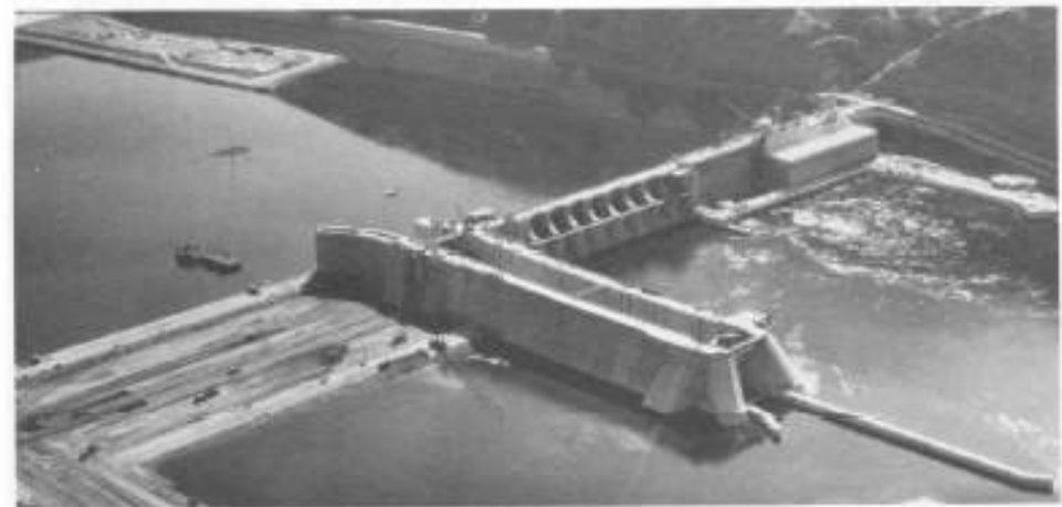
LOWER GRANITE LOCK AND DAM
