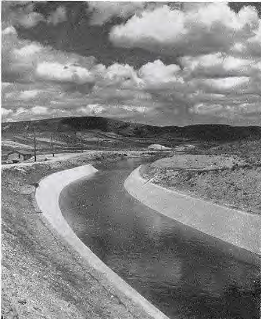
A lined canal on the Yakima project. Photo, Bureau of Reclamation.
