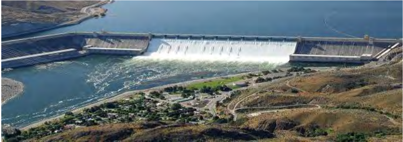
Grand Coulee Dam Aerial. Pacific Northwest Region, Bureau of Reclamation, 26 July 2017, www.usbr.gov/pn/
